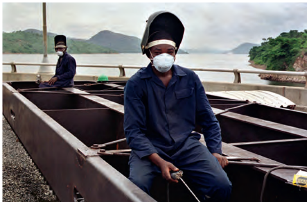
Above: Workers carry out soldering work on the Akosombo dam.
